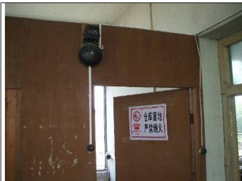
Fire alarm system were installed
