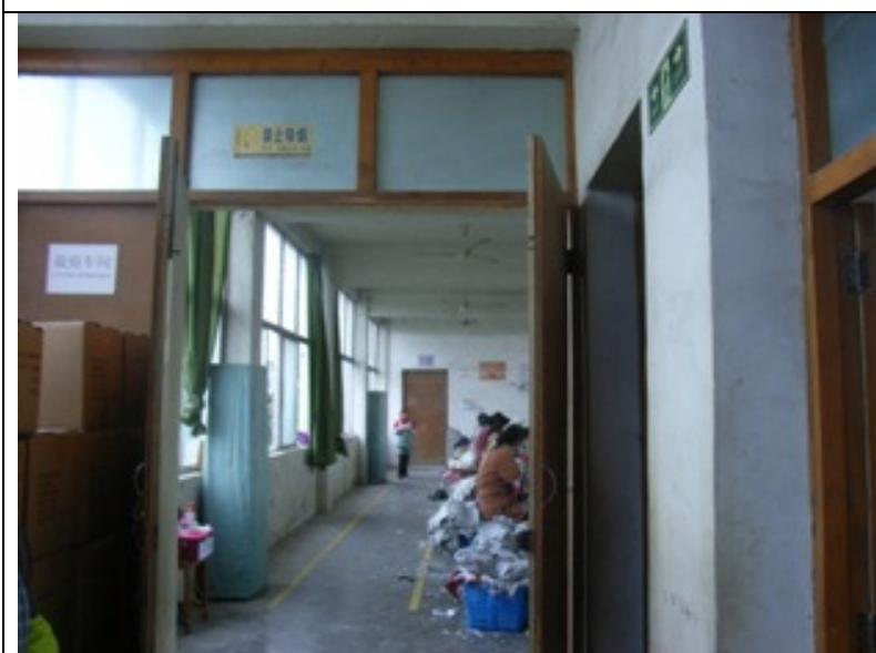
The doors of workshop were changed to open outward.
